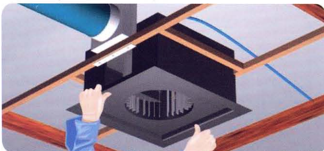
Insert housing into wood frame and tightly screw bolts.
